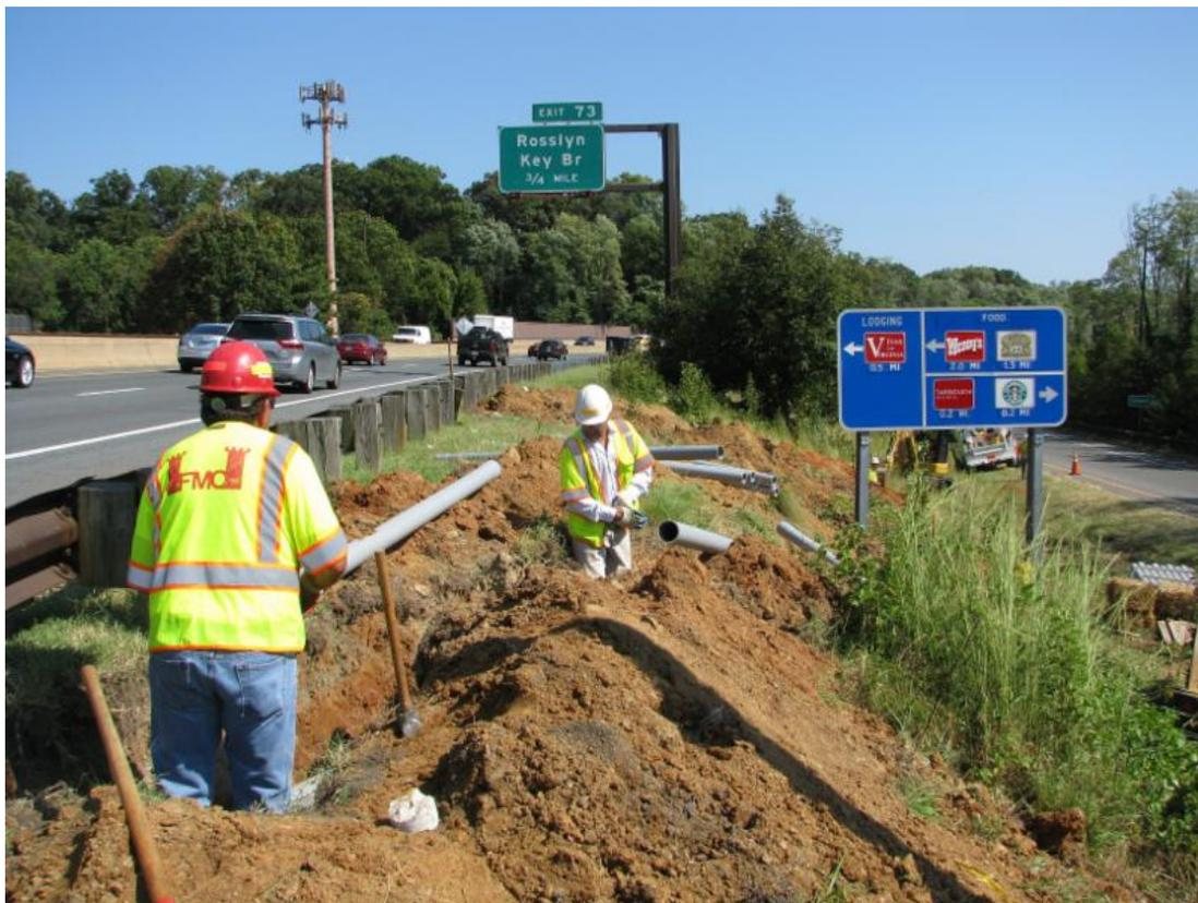
*Construction workers install electrical conduit for the rush-hour tolling system that will go into effect next year.*
